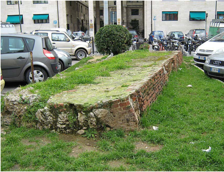
The last remaining part of Livorno's bagno complex, today in a parking lot outside the city's Government Palace (Palazzo del Governo).
